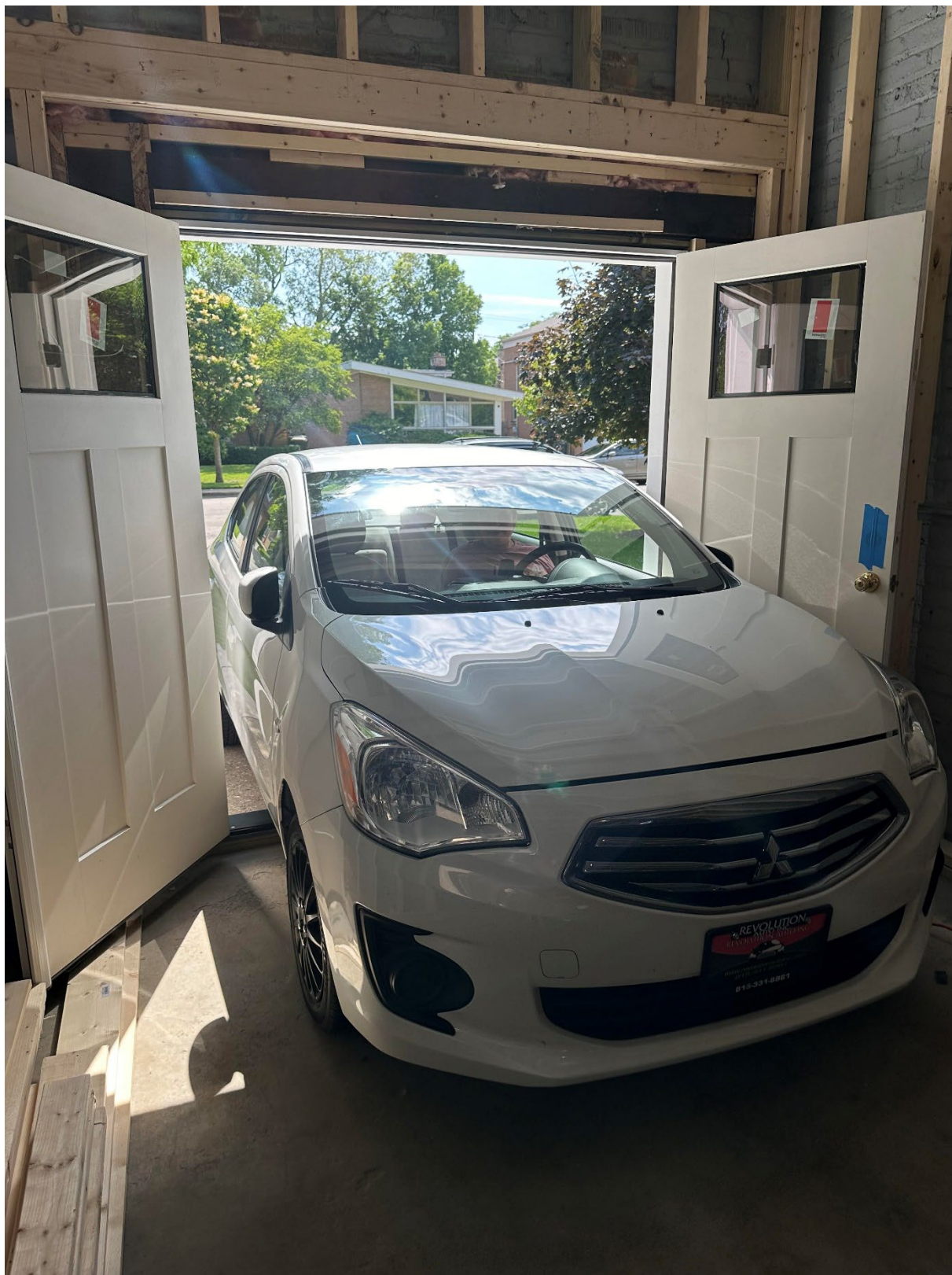
Image showing a vehicle entering the six-foot wide garage door opening
