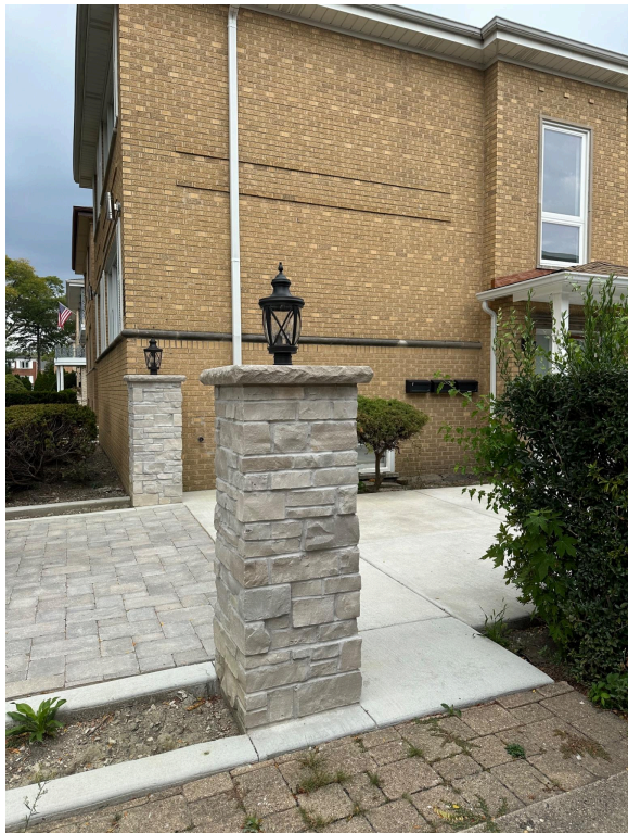
Photo of columns currently on property
