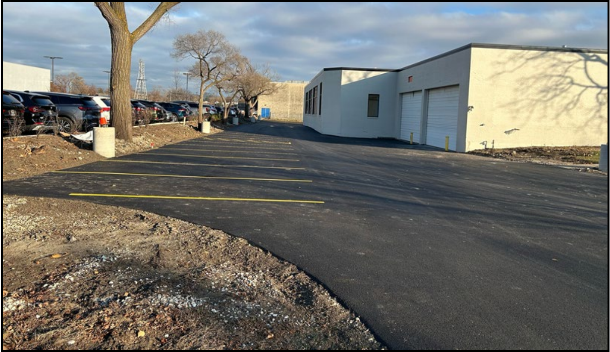
Photo of Location of North Gate (Cicero Avenue)
