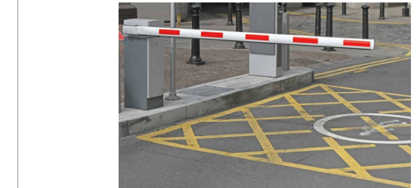
NORTH BARRIER GATE
