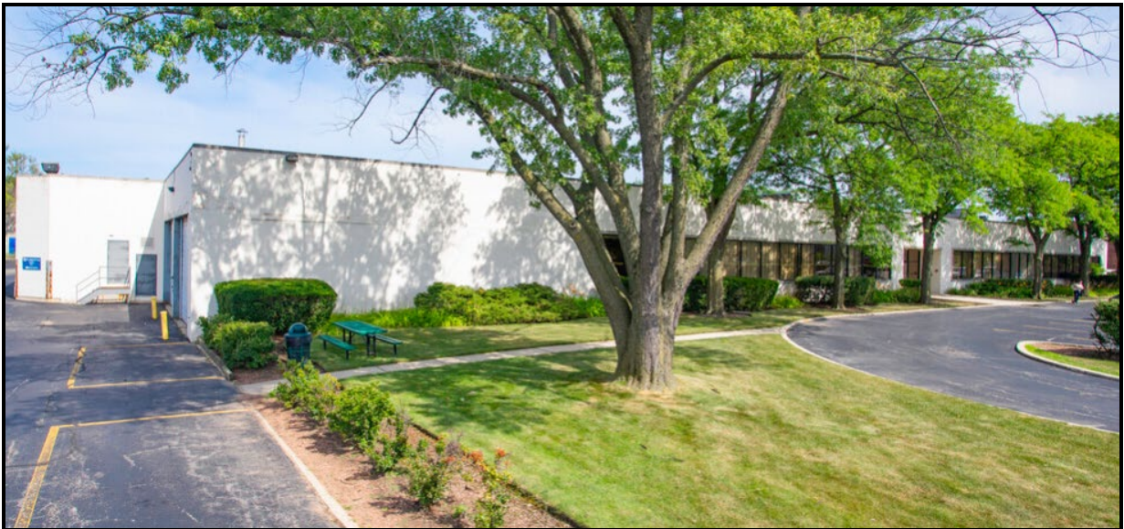
View from the Northwest Corner
